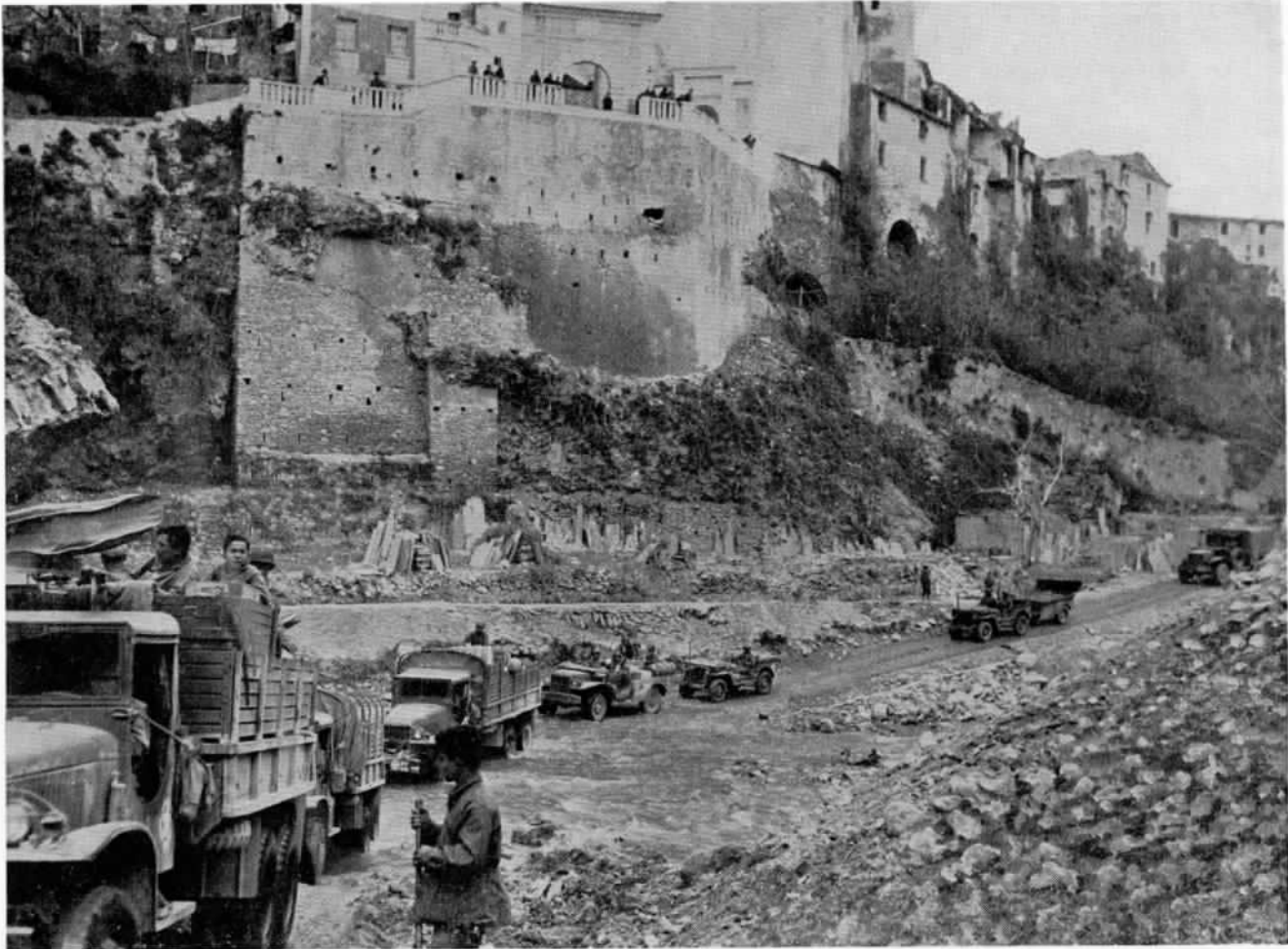
Combat Team supply convoy moves across the Frigido River over a by-pass built by the 232d Engineers
