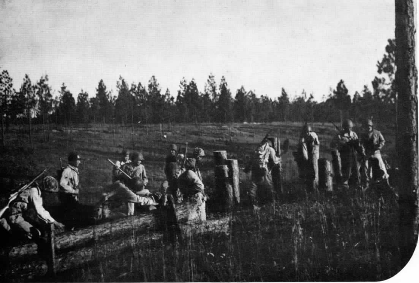
Combat engineers building tank traps.
